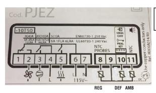
REGULATION PROBE: BLACK DEFROST PROBE: RED AMBIENT PROBE: WHITE
