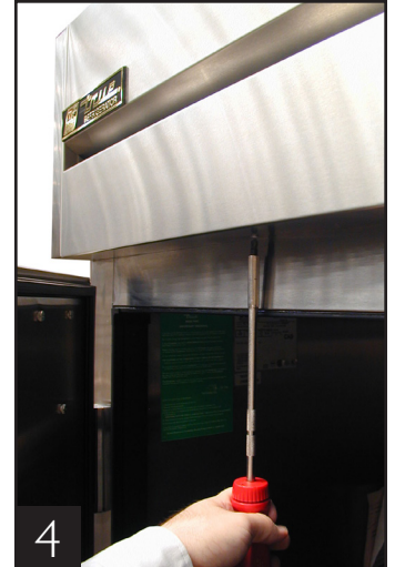
Rainshield removal, bottom screws.
