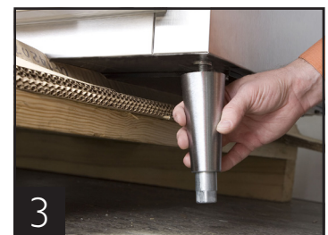
Thread leg into cabinet bottom cabinet.
