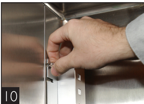
Pilaster installation (side wall of cabinet)
