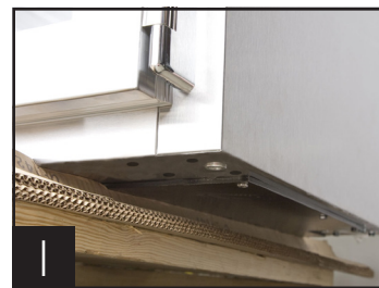
Slide packing material under the unit.
