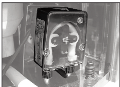
Built-in detergent and rinse chemical pumps.
